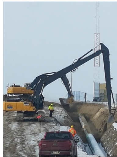
18. Shading tie-in - km 161+900 – Feb 2, 2018
