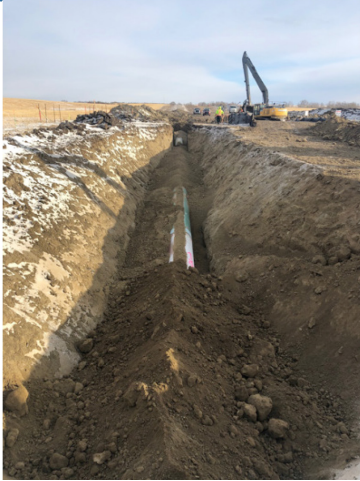
13. Backfill shading – Km 163+590 – Feb 1, 2018
