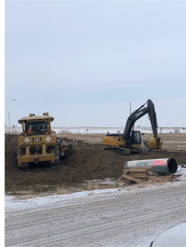
2. Backfill– km 163+500 – Jan 29, 2018
